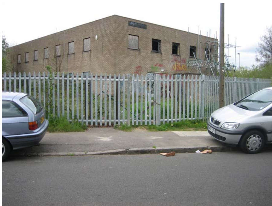
Photograph showing building from Dryfield Road
